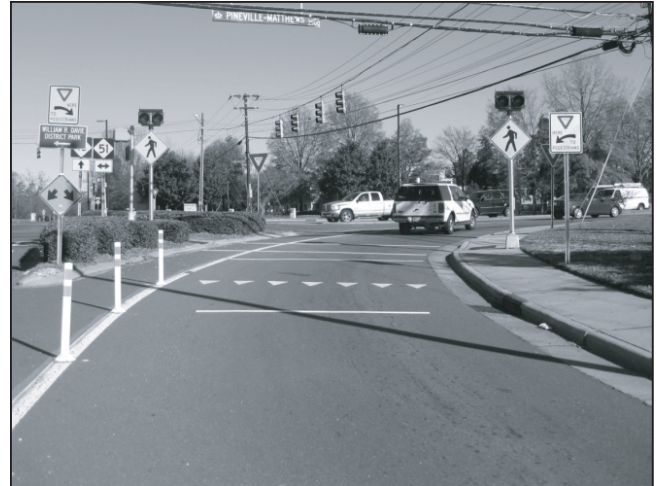
Exhibit 3. FB installation at CTL.
