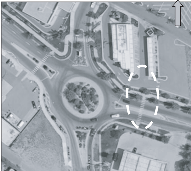
Exhibit 13. Aerial view of roundabout.
