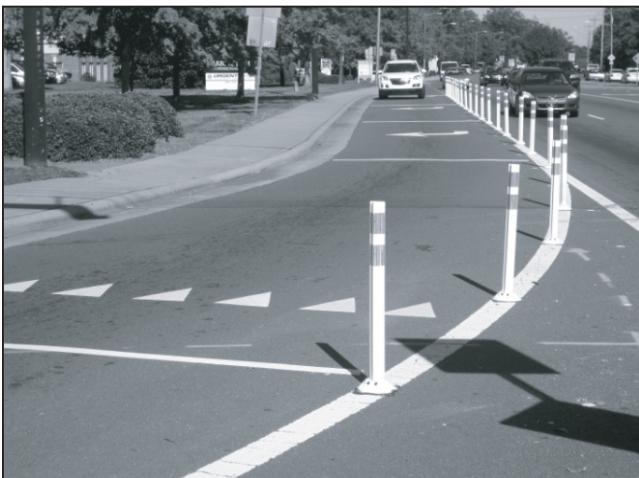
Exhibit 2. Sound strip installation at CTL.
