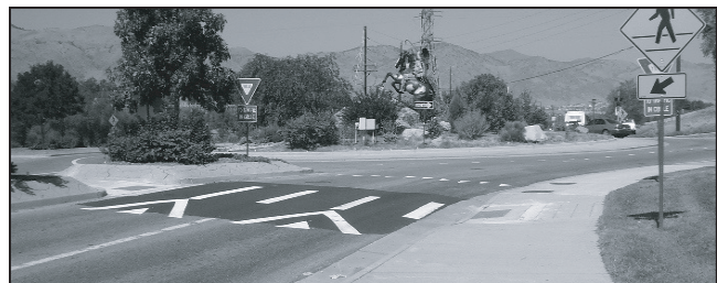
This figure shows a pedestrian-view photograph of the RCW treatment installed at the southeastern approach of the Golden Road two-lane roundabout.
